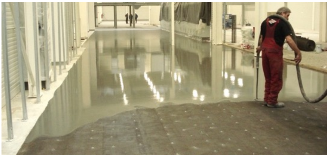
Figure 3: Mortar infiltration (left) and finished overlay (right)
