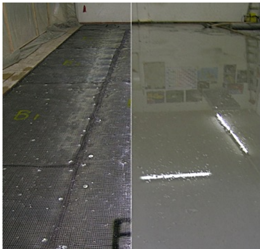
Figure 6: Manufacturing of MicroMat® and mortar infiltration (left); Burden of a DUCON surface 2 days after manufacturing by a printing machine (right)
