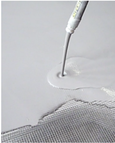
Figure 3: Mortar infiltration (left) and finished overlay (right)
