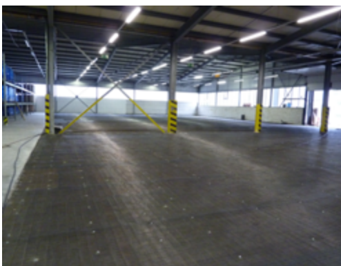
Figure 8: Overhaul (left) and completion (right) of a cracked surface with DucoPlan (d = 3 cm)
