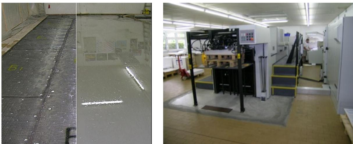
Figure 6: Manufacturing of MicroMat® and mortar infiltration (left); Burden of a DUCON surface 2 days after manufacturing by a printing machine (right)
